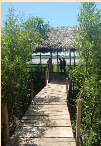
A section of the newly constructed boardwalk. Photo by Francis Kagema
