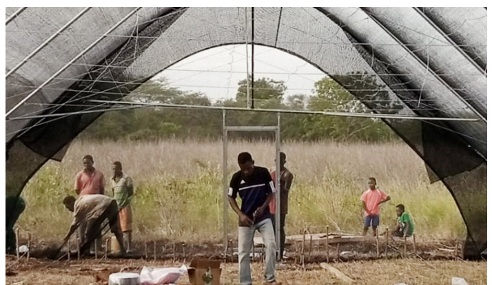
GREENING TANA DELTA: Workers install a shade house at Hewani, Tana River. The shade houses will be used for climate-smart agriculture, one of the livelihood activities aimed at increasing climate change resilience of communities at the Delta. PHOTO: BONIFACE MUSYOKA
